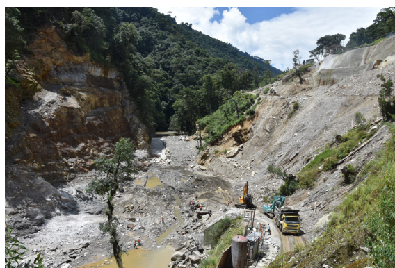
Construction of 118 MW Nikachhu Hydropower Project (Dam Excavation)
