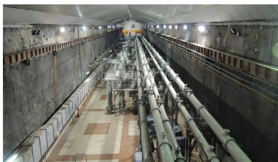
3D monitoring of GIS (Gas Insulated Switchyard) Cavern
