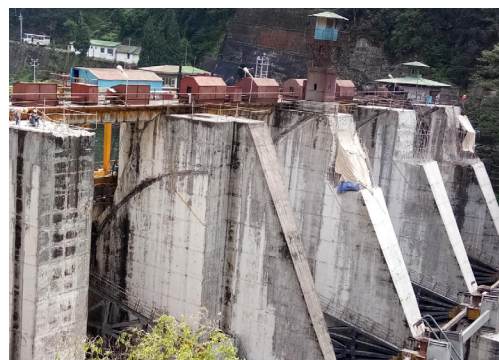
Pier cutting at Dam CHP
