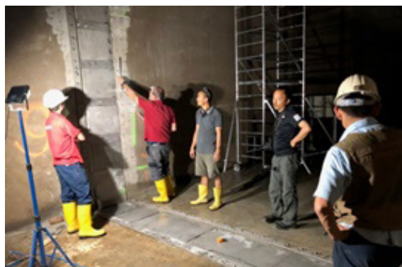
Remedial measure of HRC at Dagachhu
