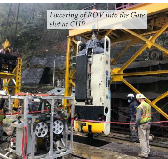
Lowering of ROV through gate slot at CHP
