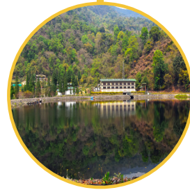
Basochhu Hydropower Plant
