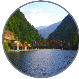
Chukha Hydropower Plant
