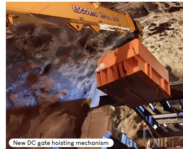
Installation of new indoor termination
