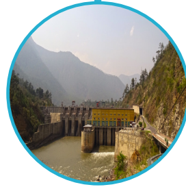
Kurichhu Hydropower Plant
