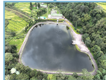
Basochhu Hydropower Plant
