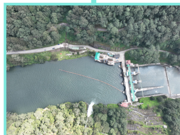
Chukha Hydropower Plant
