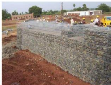
Figure 8 Lid closing procedure at site
