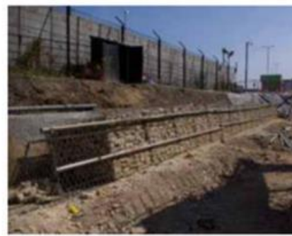
b) Use of pipes
