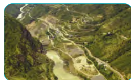
2020 Inception study on the alternative sites for the barrage/weir option for Punatsangchhu-I hydroelectric project
