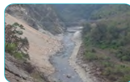
2014 Pre-feasibility study of 442 MW (125 + 317) Nyera Amari I and II integrated hydroelectric projects
