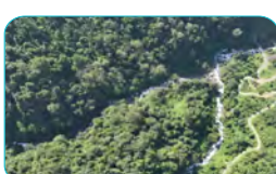
2022 Updating of Detailed Project Report of Druk Bindu I & II Small Hydropower Project
