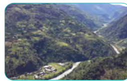
2015 - 2018 Detailed project study of 442 MW Nyera Amari I and II hydropower projects
