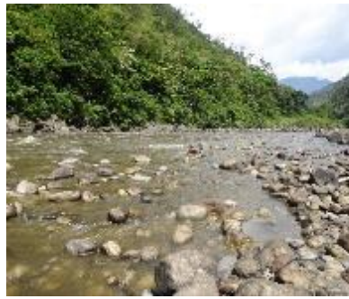
Downstream of the dam (Rewan station)
