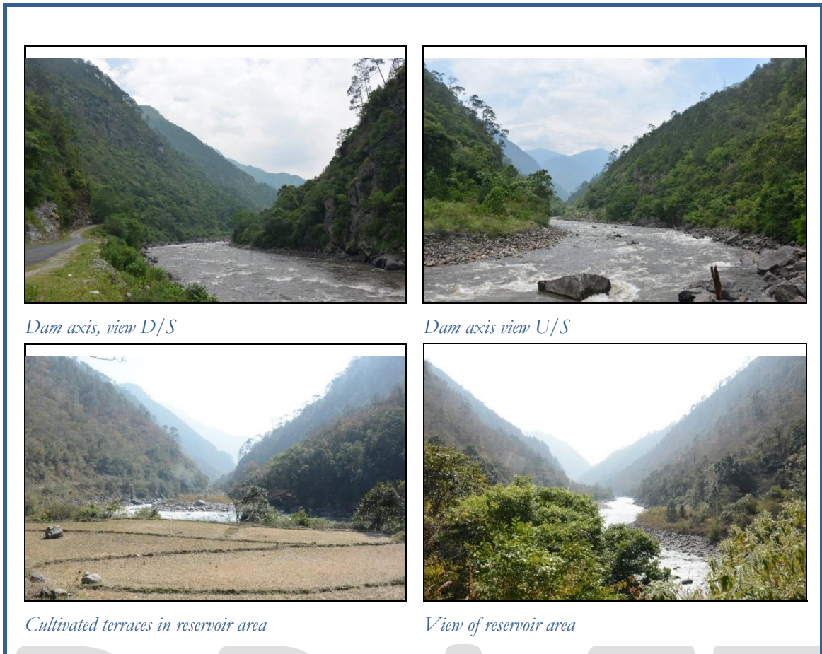
Figure 40: Photographic plate: Dam and Reservoir Area
